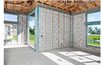
Cinder-Block Wall Construction
