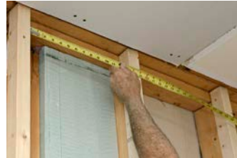
Standard 16" Stud Placement
