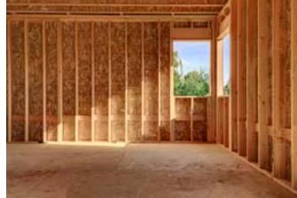
Double Wall Construction
